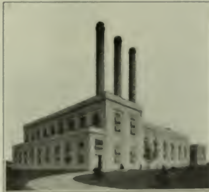
GENERATING POWER HOUSE
